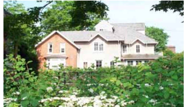
View of Rear Addition from Temperance St.
