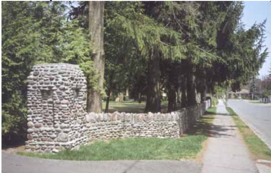
Exterior side yard stone fence/wall at 8 Beech Avenue
