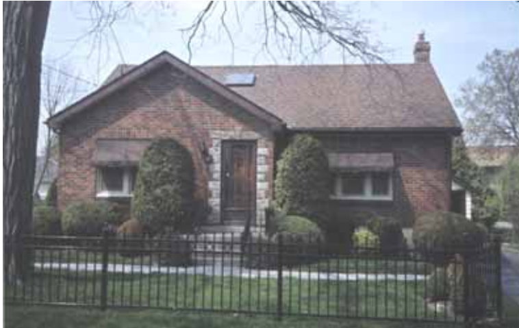
Wrought iron fence at 16 Lovers Lane
