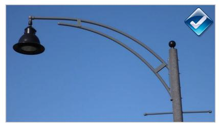
Figure 5: Full Cut-off Light Standard
