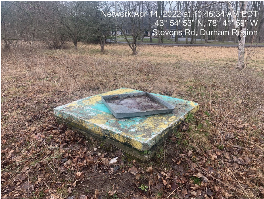
Photo 6 - View of former well on Property, facing southeast
