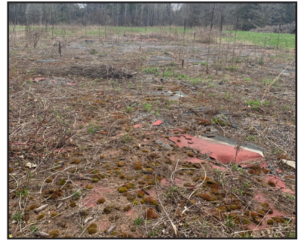
FIGURE 4.3: OLD TENNIS COURT
