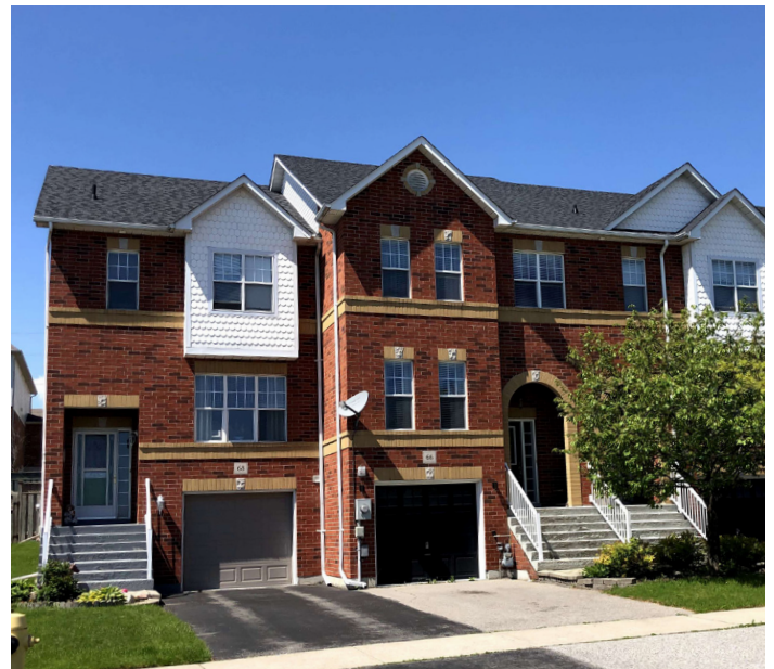
Example of existing townhouses in Bayview
