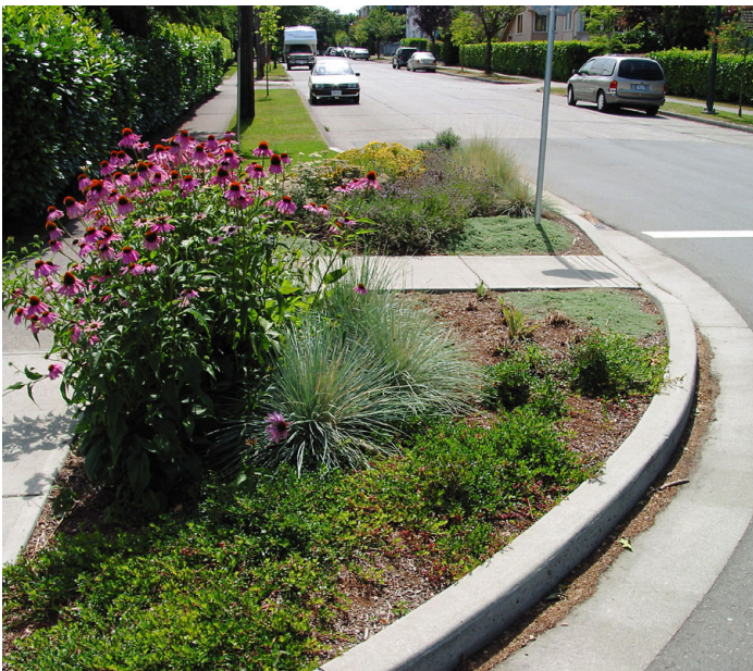
Well designed and landscaped curb extensions permit on-street parking and safe pedestrian crossings to coexist
