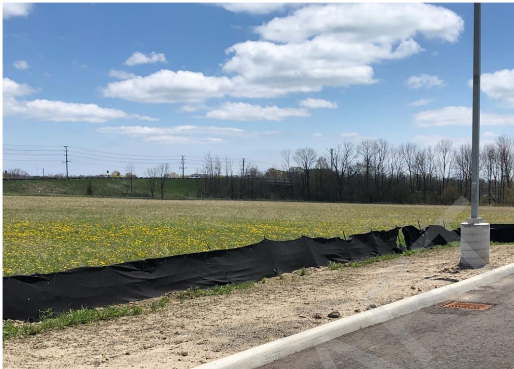
Image 22: Development and disturbance for commuter infrastructure, (Lot 29, Concession 1), view south-east
