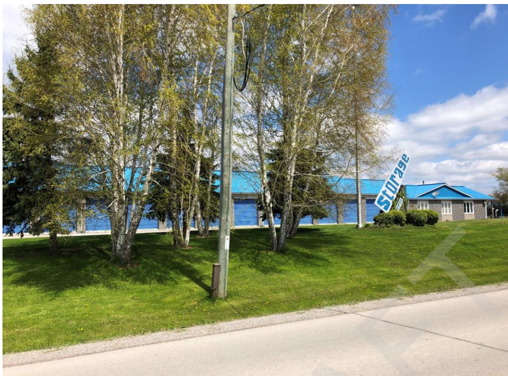
Image 14: Self storage units, disturbance due to development, infrastructure, and man-made shaping of ROW boulevard, (Baseline Road West), (Lot 31, Concession 1), view north-east
