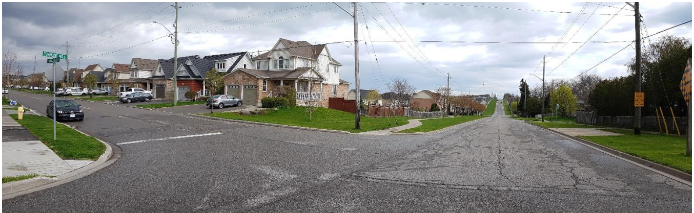
Figure 6: The intersection of Townline Road South and Gord Vinson Avenue, facing southeast.
