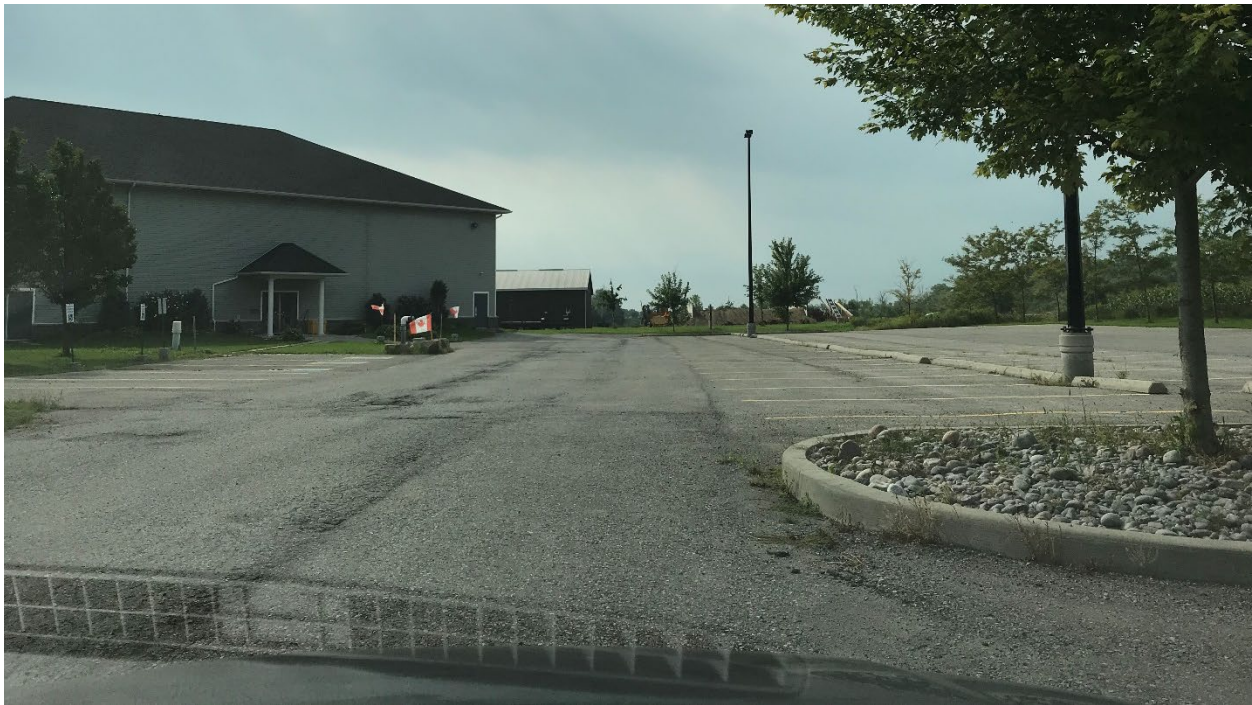
Image H-8: Example of disturbance from modern construction of a church; view south
