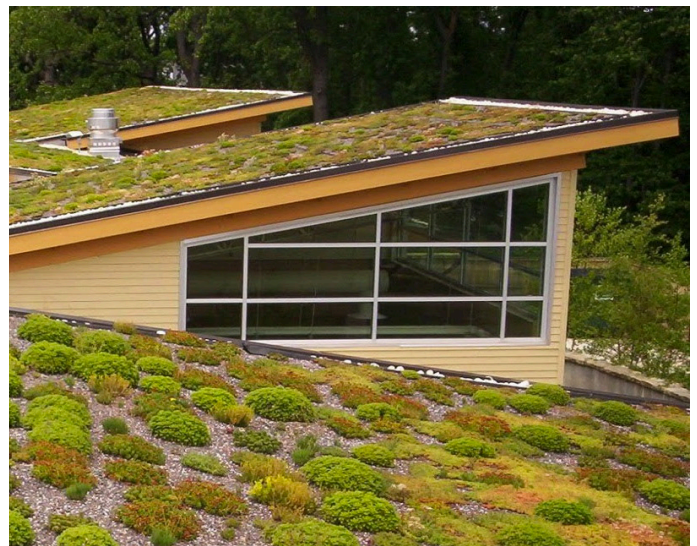
Figure 7 : Bioswales, green roofs and rain gardens are low impact development features that reduce runoff
