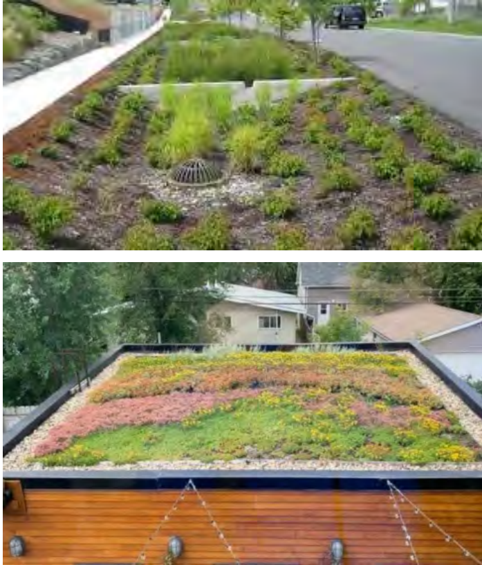
Figure 5: LIDs such as bioswales (top) and green roofs (bottom) can reduce the impacts of runoff and flooding for new developments
