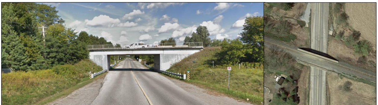
Figure 11: North Street & CP Rail Grade-Separated Crossing
