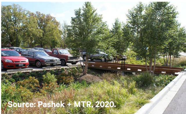
Landscaped swale for low-impact stormwater management
