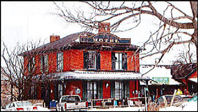
Resource No.: BHR4 - 816 Durham Road 17 Heritage Designation: Municipal Register
