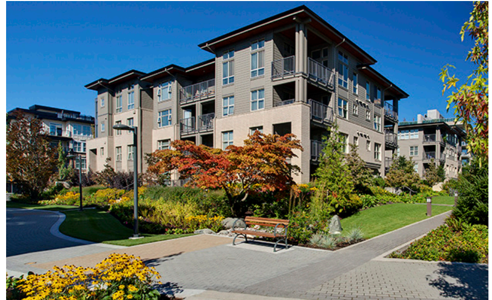
Low rise apartments (Wesbrook Village, Vancouver)
