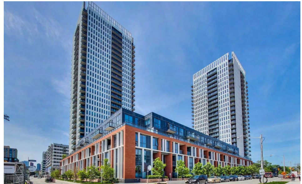
Towers on a low-rise, mixed use podium (Regent Park, Toronto)
