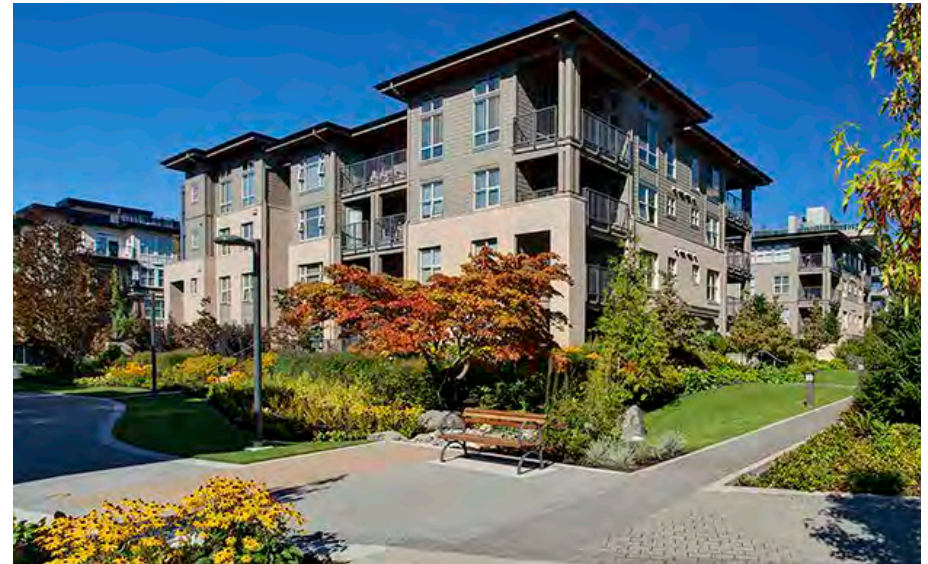
Low rise apartments (Wesbrook Village, Vancouver)
