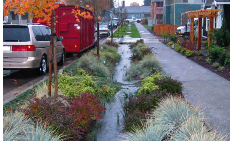
Low-impact development stormwater management
