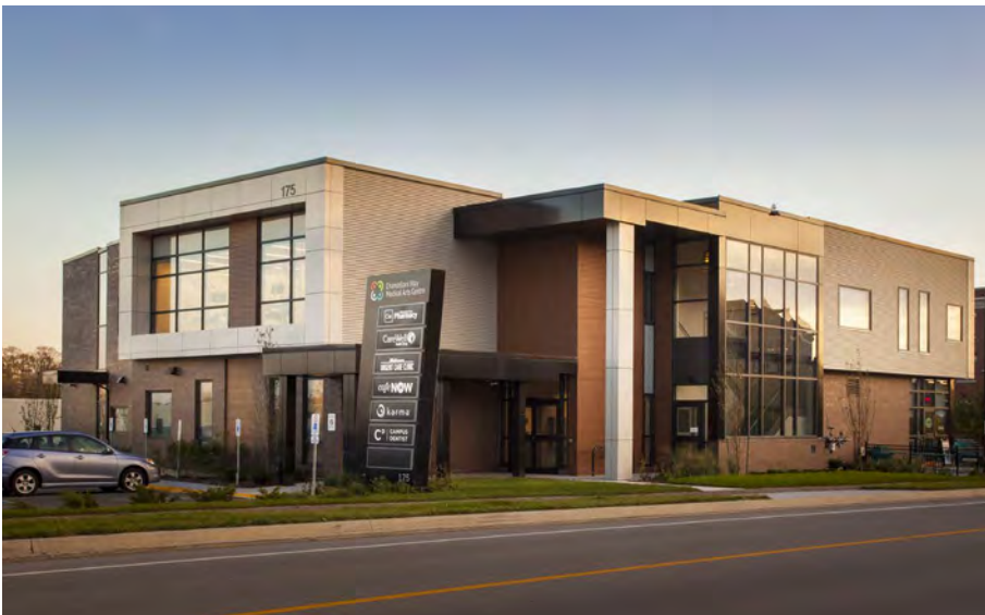
Small service offices (Medical Arts Centre, Guelph)
