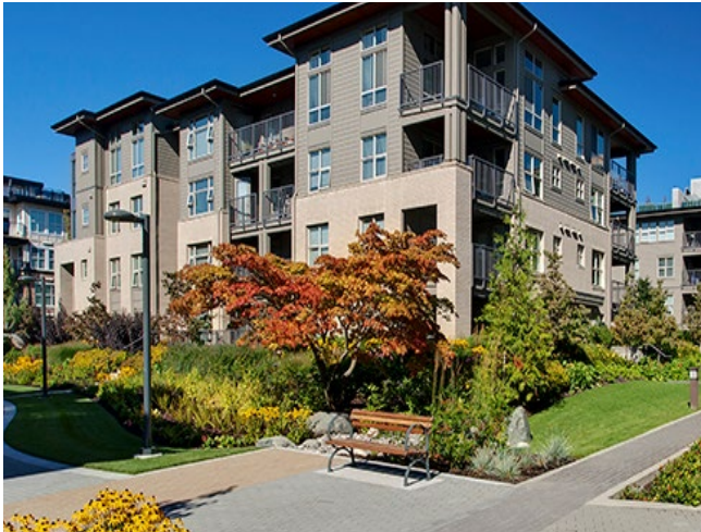
Low-rise apartments (Wesbrook Village, Vancouver)
