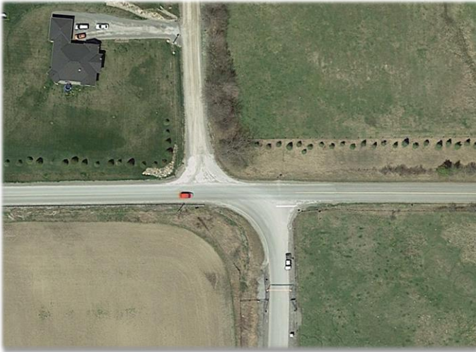
Aerial Image of the Concession Road 1 and Elliott Road Intersection – Google Earth Imagery 2018
