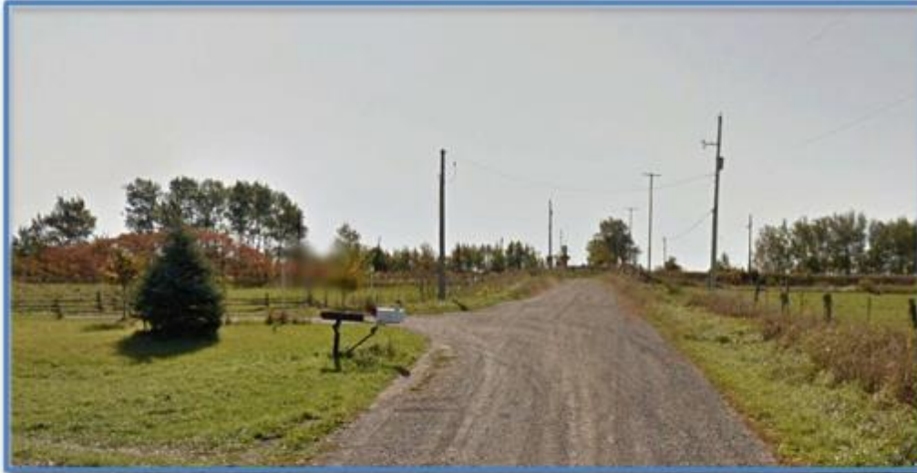
Nichols Road approaching the existing rail crossing looking South – Google Imagery 2011
