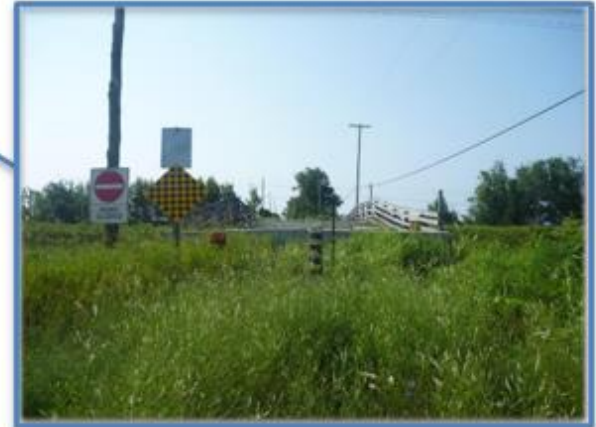
Nichols Road at rail crossing looking South – 2014
