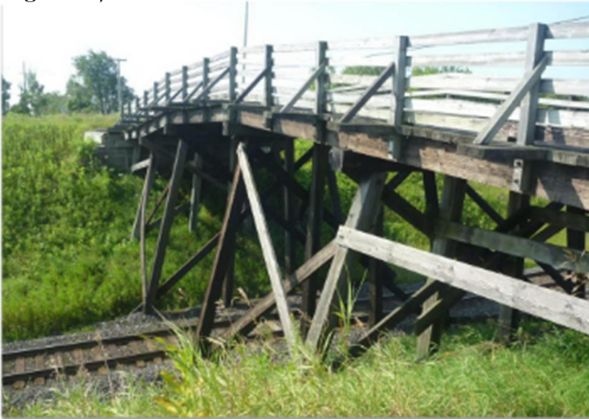
Nichols Road rail crossing east elevation – 2014
